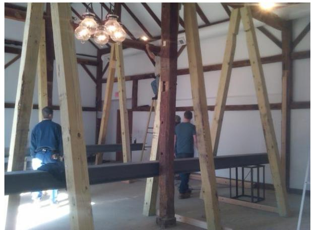
*Temporary posts were used to prop up the weight of the White Barn before the steel beams (the long horizontal gray I-beams in the photo) were installed. Photo by Laura Way*
